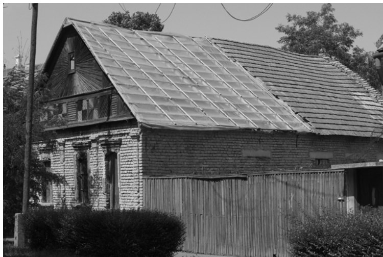
Figure 2.: Ruined house with sunbeam gable (Szeged-Uppertown)
